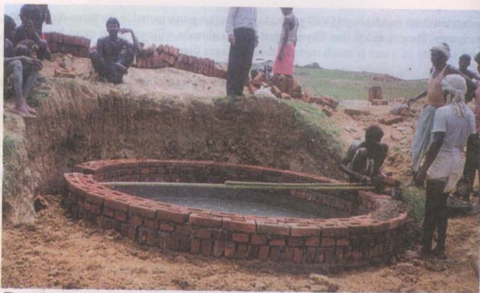
The artisan well at Shyاملapur nearing completion
